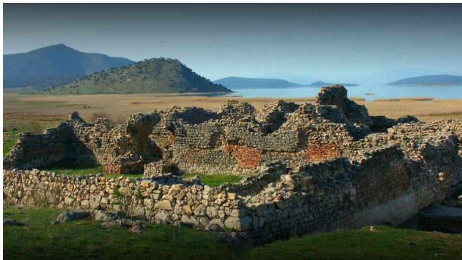
Figure 6. A general view of the walls today [40].
