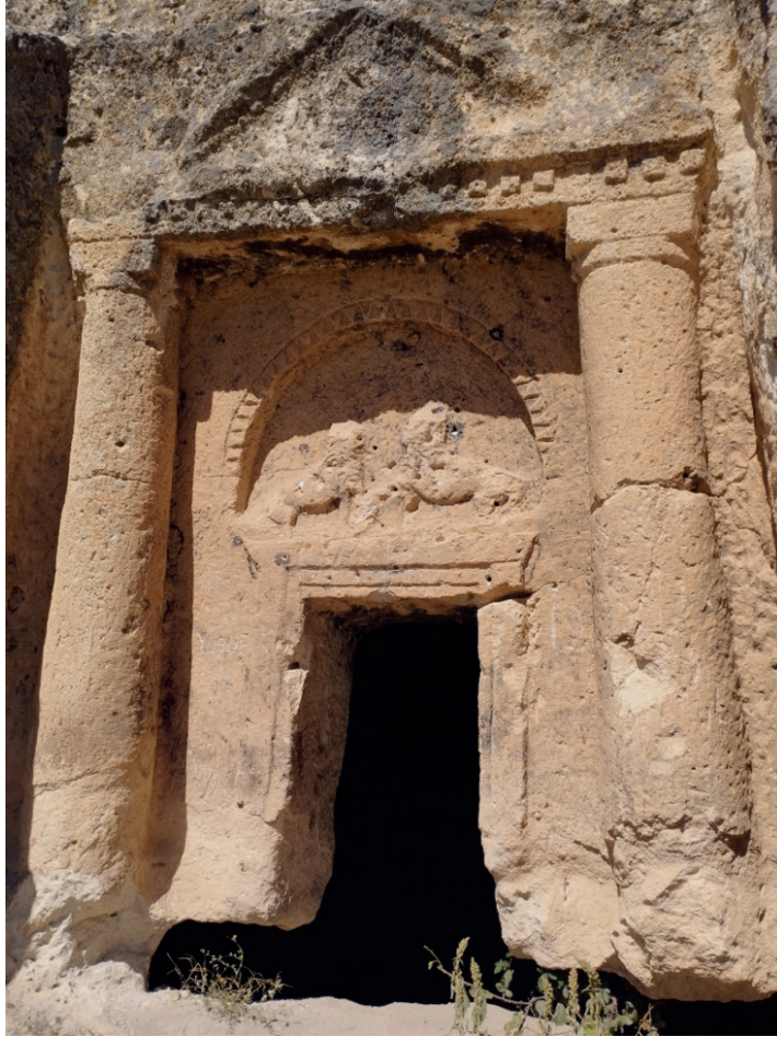
Figure 3. Missing Part Anomaly
