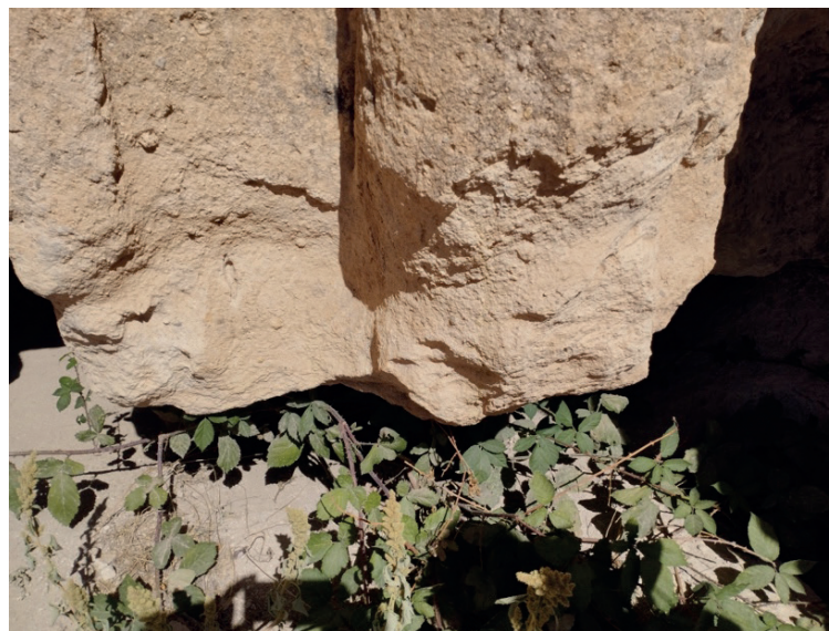
Figure 2. Contour Scaling With The Maximum Depth Observed On The Monument
