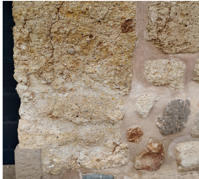
Figure 9. Differential erosion caused by matrix loss
