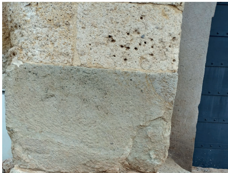
Figure 8. Contour scaling development
