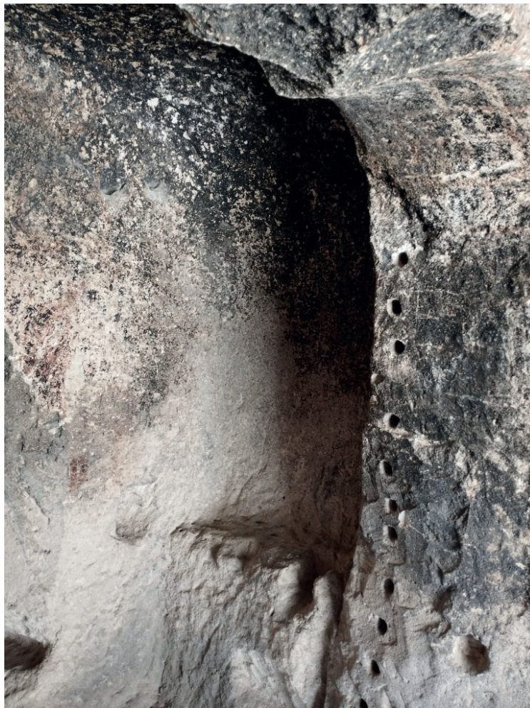
Figure 3. Black crust observed in the church
