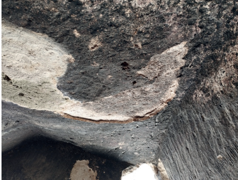
Figure 2. Contour scaling and black crust on the monument ceiling
