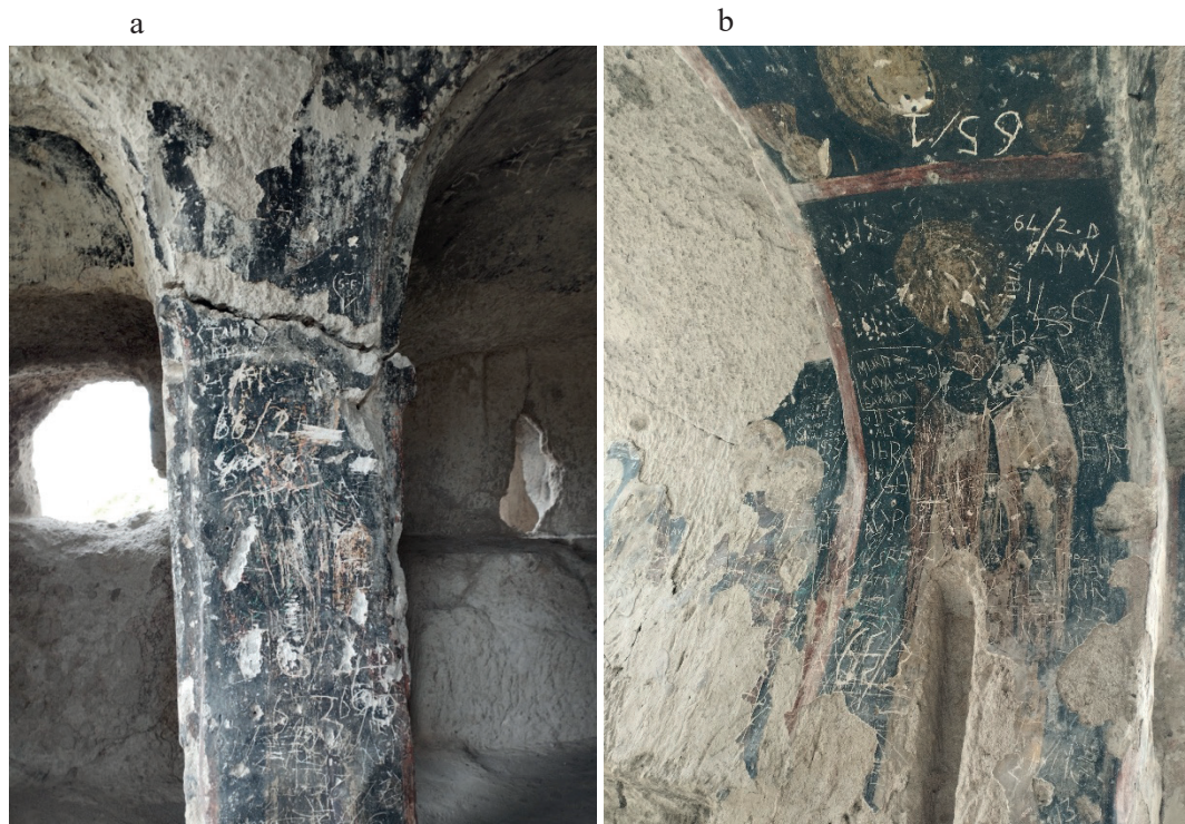
Figure 6. a) Loss of fresco, graffiti, and crack detected in the structural system of the monument, b) Loss of fresco and graffiti observed on the wall
