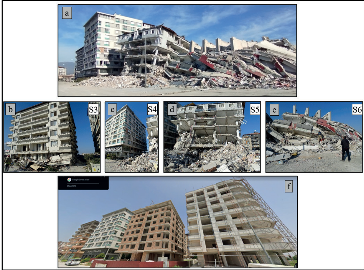
Figure 3. a) View of buildings with different types of damage on Atatürk caddesinde (location 2), b) Building 3 (S3), c) Building 4 (S4), d) Building 5 (S5), e) Building 6 (S6), f) Google.maps image of buildings before earthquake ( https://www.google.com.tr/maps/ )
