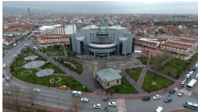
Figure 8. Karatay Town Hall Built in Place of Traditional Housing Fabric
