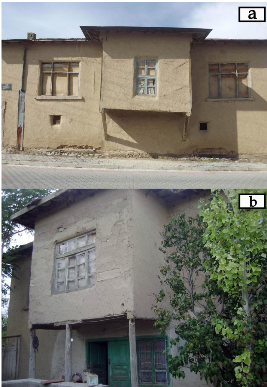
Figure 5. "Cumba" forms in houses with code number Sry-001 and Sry-016, whose plan schemes are presented in Fig 4
