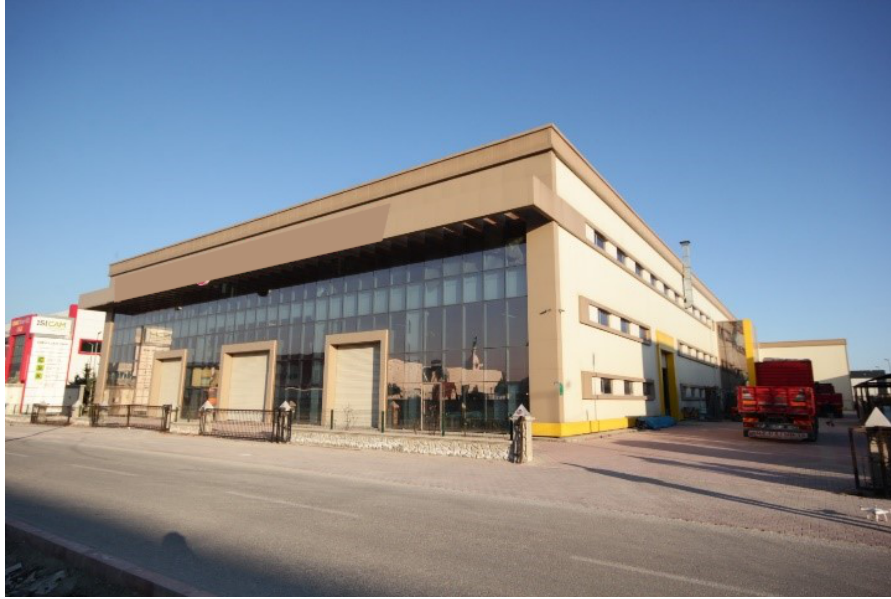
Figure 3: Facade of glass factory.
