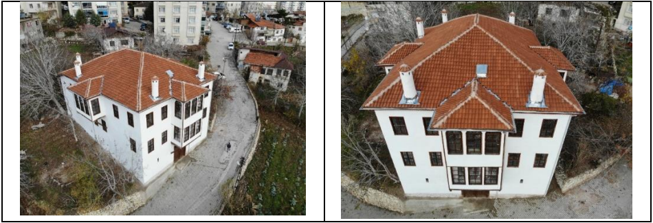
Figure 6. Photos of historical building after the insulation retrofitting.
