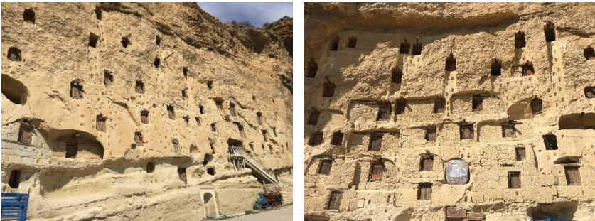
Figure 12. Grain Silos (Personal archive, 2023)
