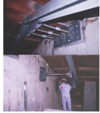
Figure 7. The Basilica of San Francesco and the usage of SMA on the roof (Castellano et al., 2001; Ytur, 2023)
