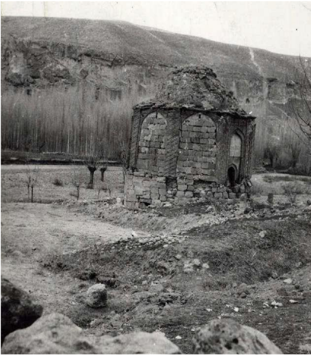
Figure 5. Structural deformations of Tomb around 60's.
