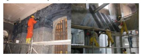
Figure 7. Reinforcement with fibre reinforced composites in historical buildings, Source: Peker, 2005.
