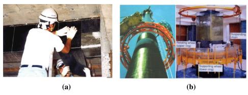
**Figure 2.** (a) Fibrous polymer application in beams, (b) Fibrous polymer application in columns, **Source:** Canbay, 2020.
