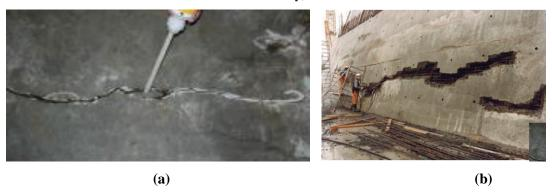
**Figure 3.** (a) Reinforcement application with epoxy resins, (b) Reinforcement application with repair mortar, **Source:** Canbay, 2020.
