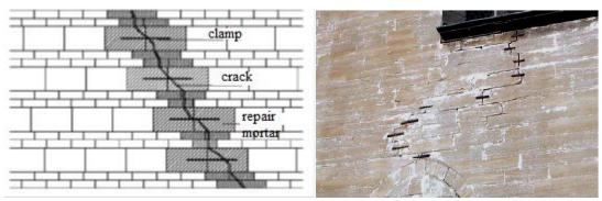
Figure 8. Repairing wide cracks by sewing, Source: Aköz, 2008.
