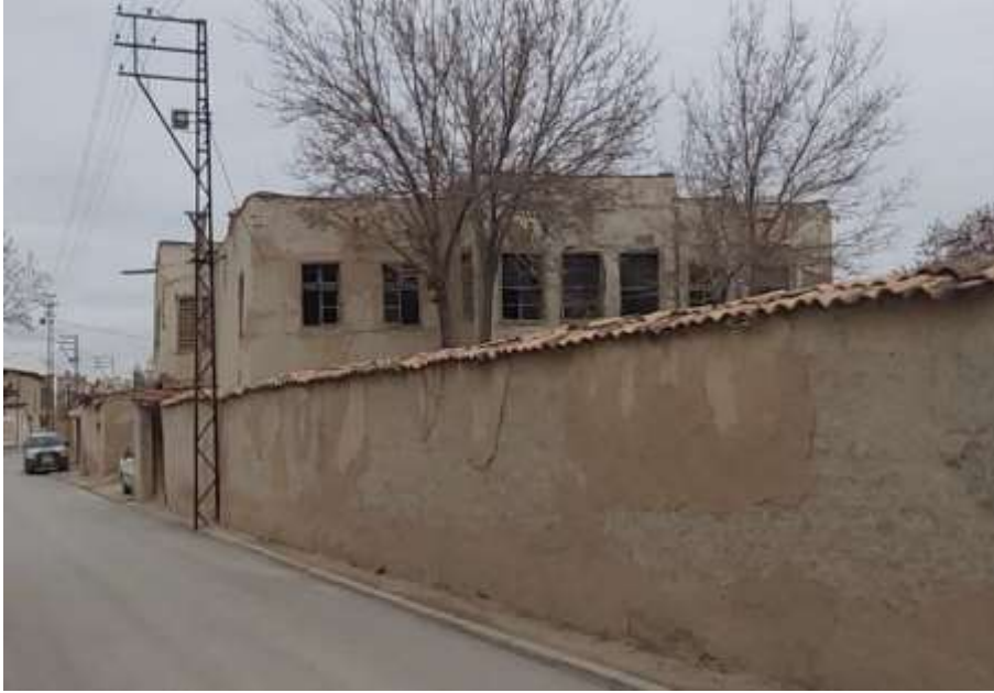
Figure 2. Nakipoğlu House Facade (Dönmez, 2021)
