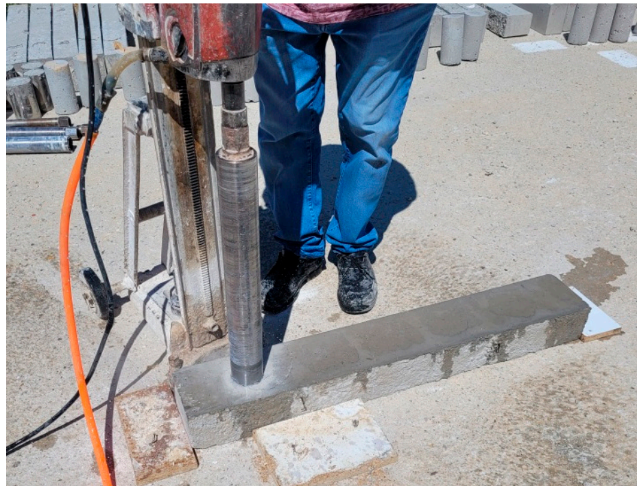
Figure 1. Preparation of beams with circular openings.
