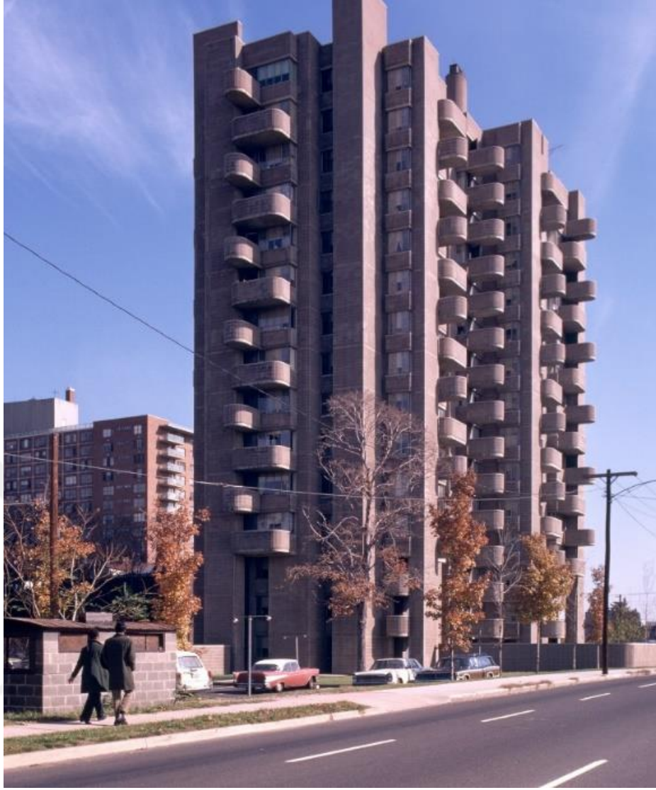
Şekil 3.32. Crawford Manor, Paul Rudolph, 1966, New Haven/ABD (URL 36)
