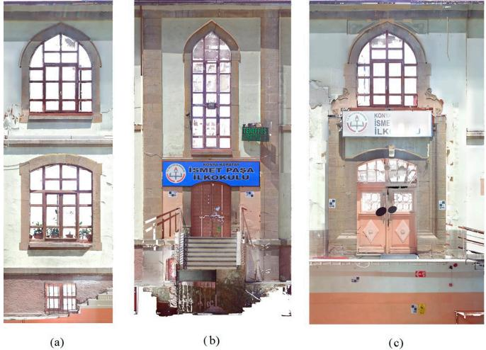
**Figure 9.** Orthophotos acquired from the point cloud with As-Built software: (**a**) windows; (**b**) back door and vertical window; and (**c**) front door and window.
