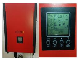
Figure 8. 3 Phase Hybrid Inverter
