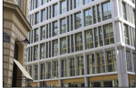
Şekil 2.75. Le Bon Coin (HeidelbergCement Group, 2022b)
