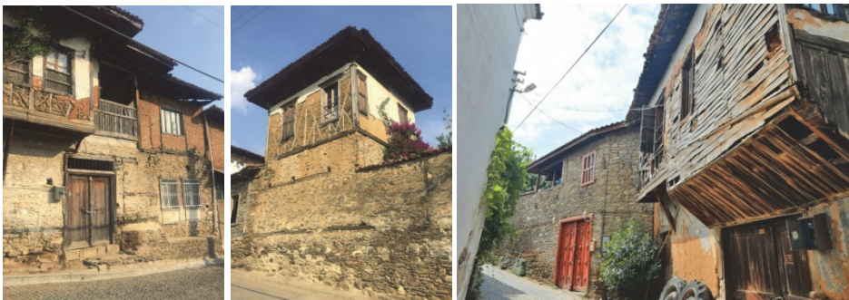
Restoration of a local construction in Birgi (Genç, 2019)
