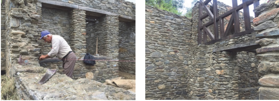
Restoration of a traditional house in Birgi (Genç, 2019)
