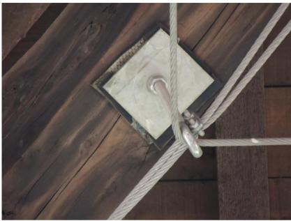
**Figure 3.** A detail of the wood beam reinforcement of the roof of one tower of Pavia Castle, Italy. The new addition is completely reversible. Project: Lorenzo Jurina (photo: Andrea L'Erario, 2014)
