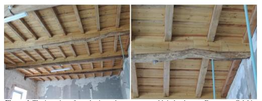
**Figure 4.** The insertion of new horizontal structures on old timber beams, Ex caserca Calchi, Pavia, Italy. The historical beams are reinforced by the addition of new beams (photo: Andrea L'Erario, 2014)
