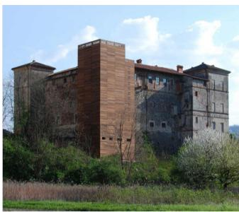
**Figure 5.** Saliceto Castle, Italy. Restoration project by Armellino&Poggio Architetti Associati, 2011. The new tower, made with a steel and timber cladding self-supporting structure, is well noticeable from the historic castle.
