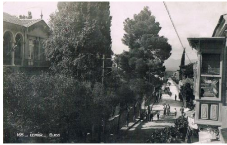
Figure 6. Station Street (Uğur Mumcu St)
