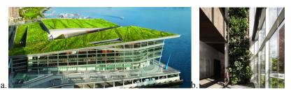
Figure 5: a. Green roof of the Vancouver Convention Center (Canada, 2009), b. Atrium with living wall [21, 22]
