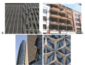
Figure 6: Computerized panels : a. Kinetic façade b. ThyssenKrupp Quarter Essen Building (Germany, 2010) façade, [23-25], c. Al Bahar Tower, overall view from the north and folded panel view
