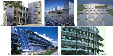
Figure 4: Building-integrated photovoltaics (BIPV) in the façade and roof [16-20] :
