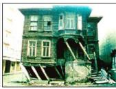
Figure 1. Earthquake damage for masonry and timber structures (Prohitech 2004)
