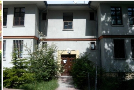
Figure 9. Façade and front yard
