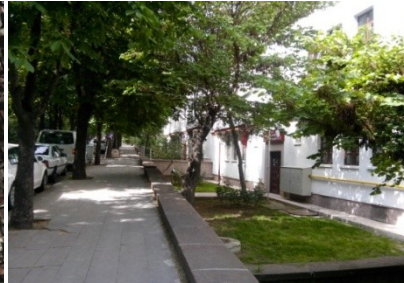
Figure 7. Building, yard and sidewalk
