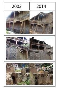
exposed after the surface brickwork has shed. Rain and wind will deprive the load-bearing capacity of the
