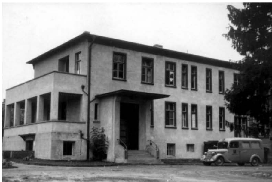
Figure 2. The 1930s modernization and extension. Photo courtesy: dr Justyna Liguz
