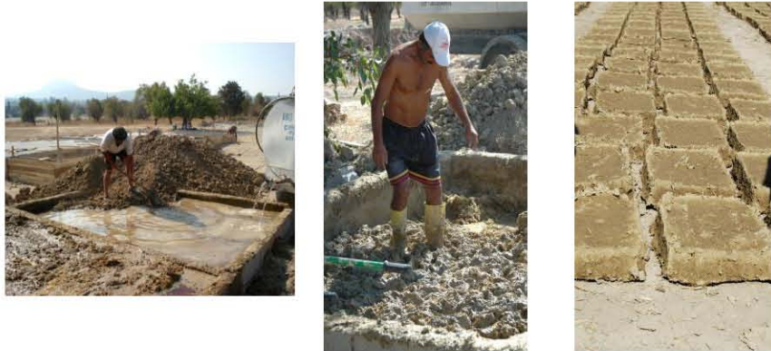
Figure 7. Preparation of mud brick [Özbekoğlu 2008]
