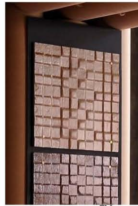
Figure 5. Strawave™ applied as inner cladding, out of rice straw and uncolored conventional epoxy resin.
